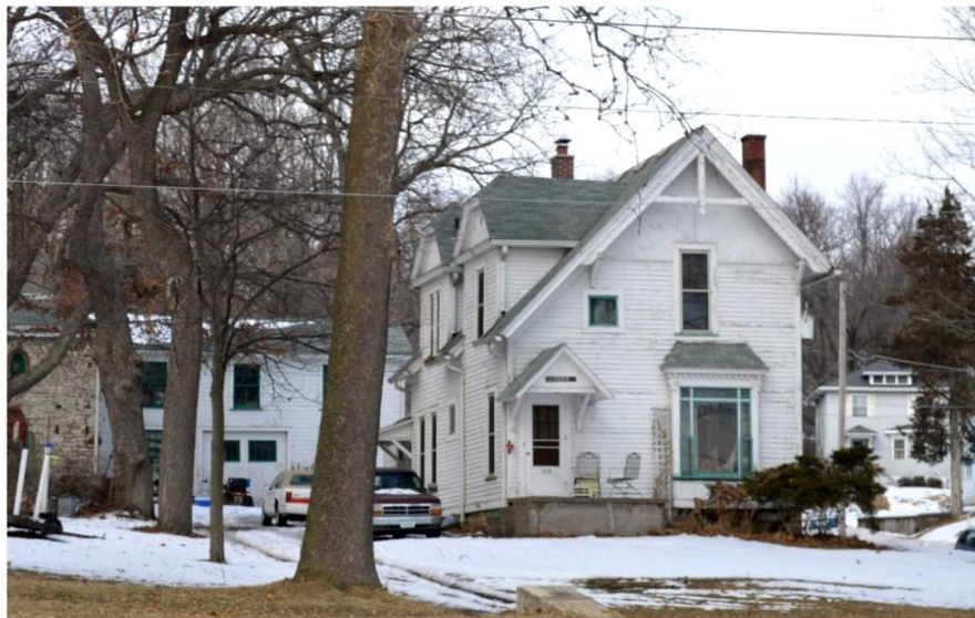
Figure 83 The C. J. Von Maur House c 1875, 1326 East River Drive. This property and the Nutting Carriage Barn have the same address, with the barn at the rear. Source: Author photo, 2/6/2015
