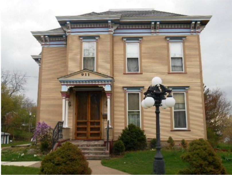
Figure 58 The James E. Lindsay House c 1876. Davenport, Iowa. Italianate in wood clapboard. Source: Scott County Iowa Assessor, = http://parcels.scottcountyiowa.com/pmc/daven-
