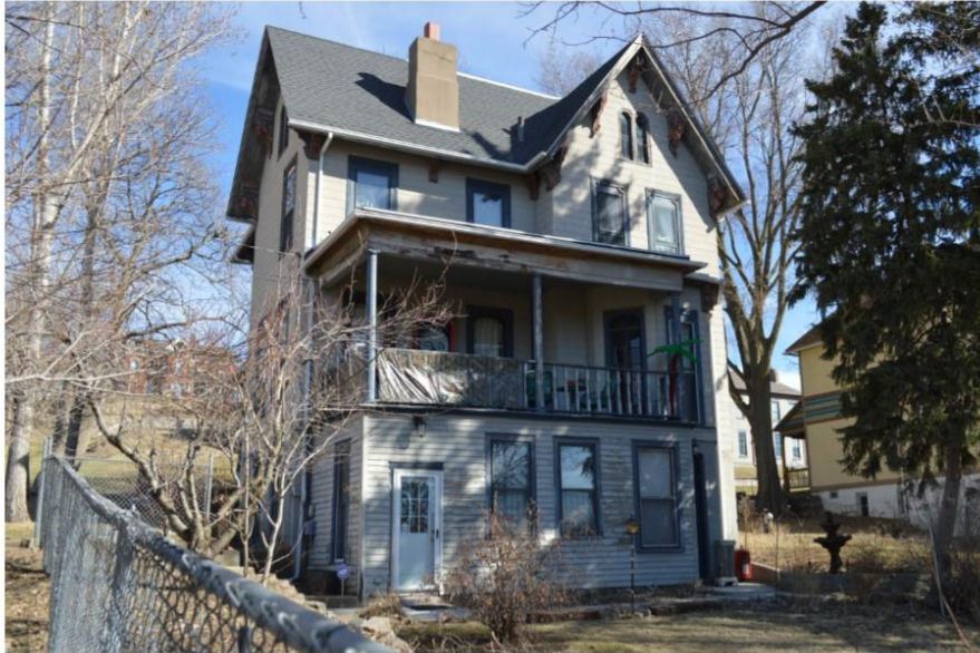
Figure 44 Francis Ochs House looking NE at south elevation. House takes advantage of its site. Locally called a "Davenport Two-and-a-Half" for the varying number of stories exposed. Source: Author photograph, 3/17/2015
