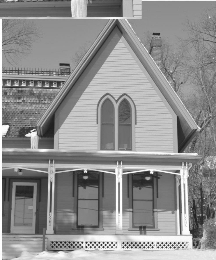
Figure 11 William Foster House 2/4/2015 South façade showing de- tail of lancet windows, gable trim and porch Source: Author Photos
