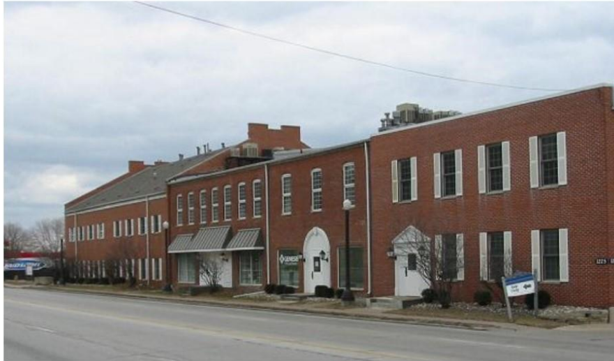
Figure 84 The Shields Woolen Mill c 1863-68, 1225 East River Drive. Source: Scott County Assessor's website information for 1225 East River Drive.
