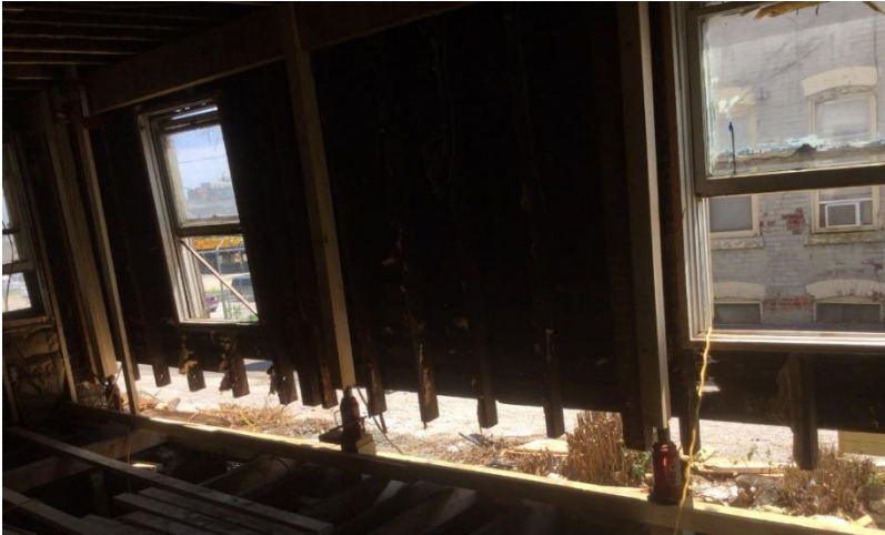
Figure 4 Looking southeast, south wall lifted for new sill, studs trimmed of rotted material and awaiting butt joining with good wood and sistered before being lowered into place. 7/14/2016 GRG photo; used with permission.
