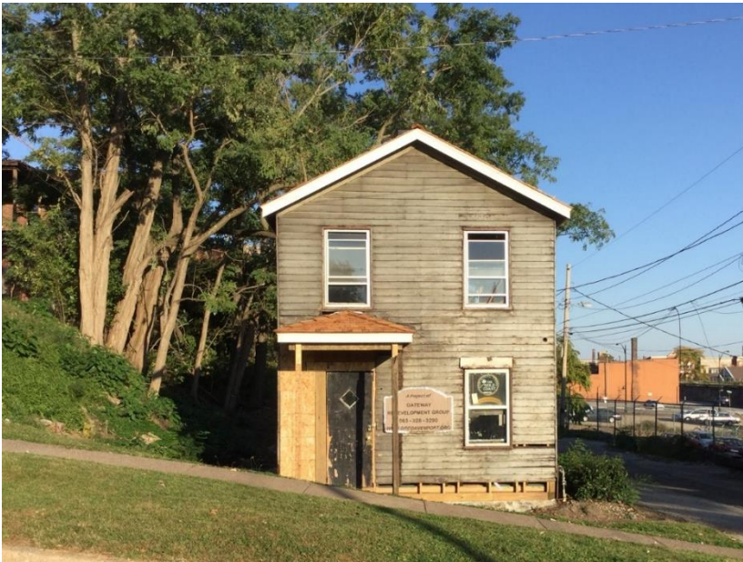
Figure 6 Looking east, Cottage after remediation to sills, new roof and removal of later cladding. 10/11/2016 GRG photo; used with permission.
