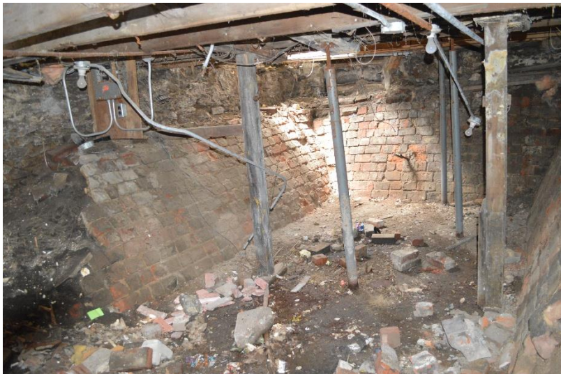
Figure 3 Looking southwest, battered brick walls in basement below limestone foundation. 5/25/2016 Author photo.
