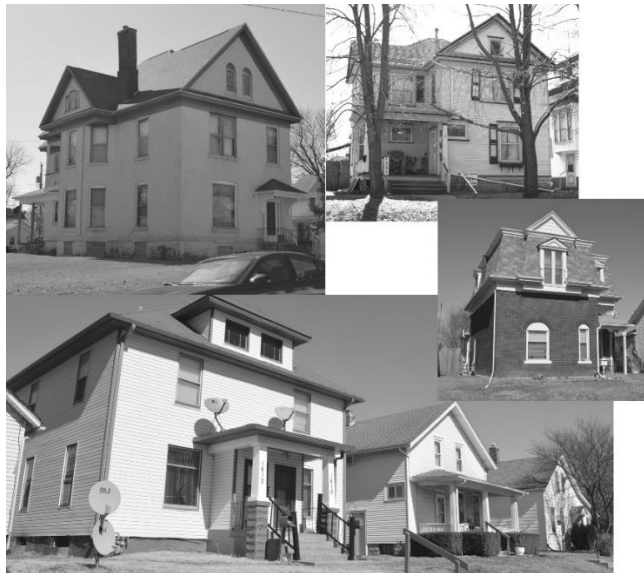
Figure 8: Houses along West 13 th Street. A variety of types; houses in bottom photo have all had original cladding covered or replaced with modern vinyl or metal. [Source: Author photographs, March 1, 2018.]
